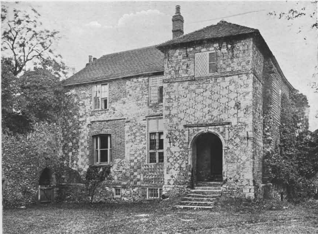
LOT 17.—ST. RADEGUND'S ABBEY. THE FARMHOUSE SHOWING THE XVI. CENTURY FLINT CHEQUER-WORK.
