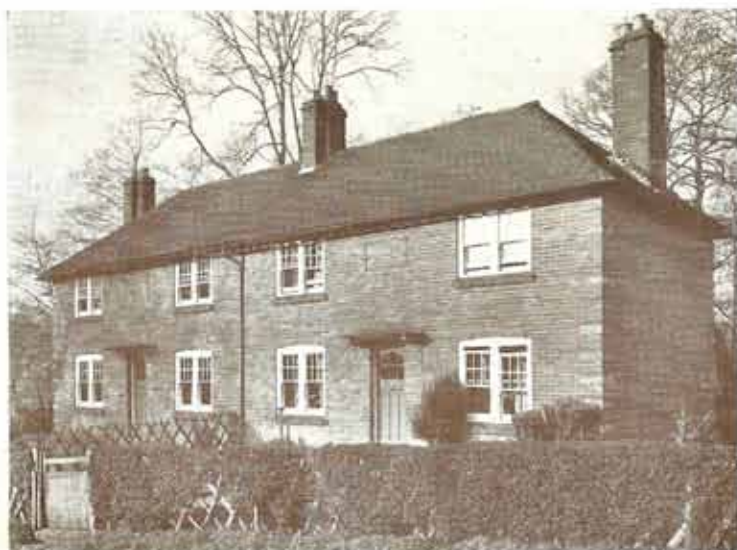
Lots 23 and 24 Nos. 1 and 2 HURSTFORD LANE COTTAGES
