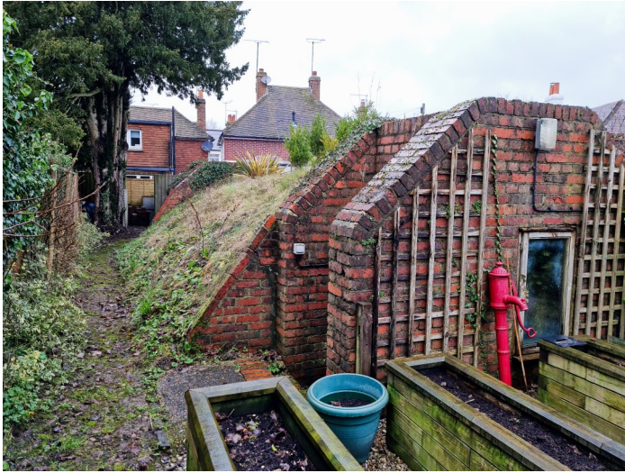
Our air raid shelter
