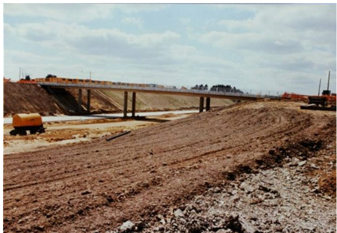
Pluckley Road Bridge under construction
