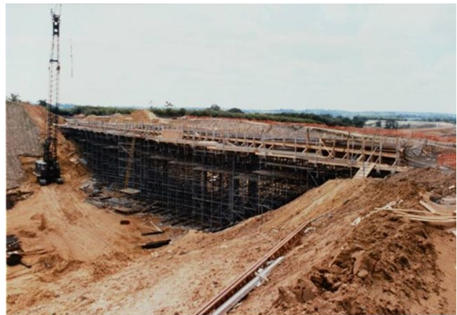
A20 /M20 Bridge under construction at Westwell
