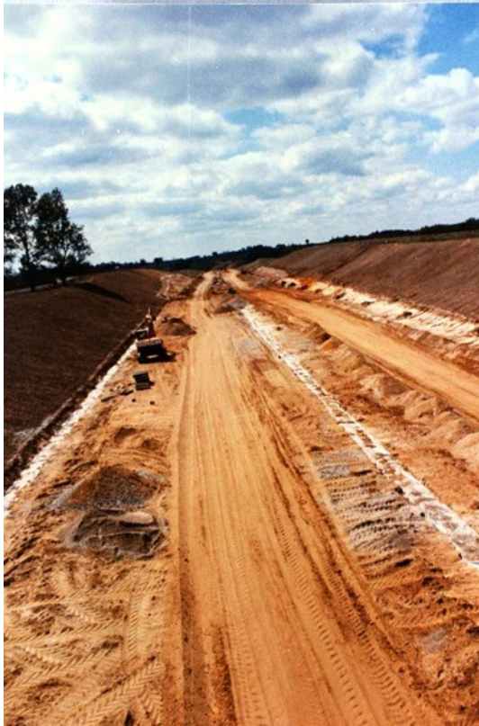
Section around Charing still under construction
